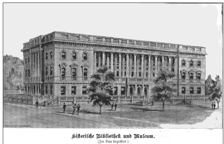
The “Historical Library and Museum,” under construction
