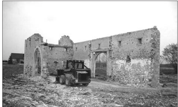
Dismantling the Mamer/Hansen barn.
